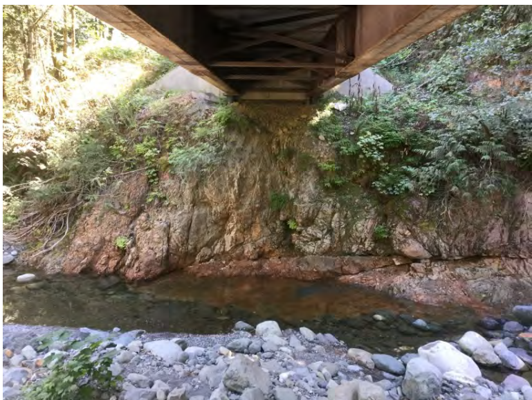
Right Bank Abutment when facing downstream
