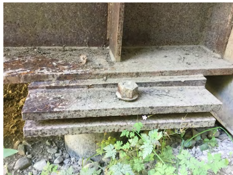
Bearing shim - typical
