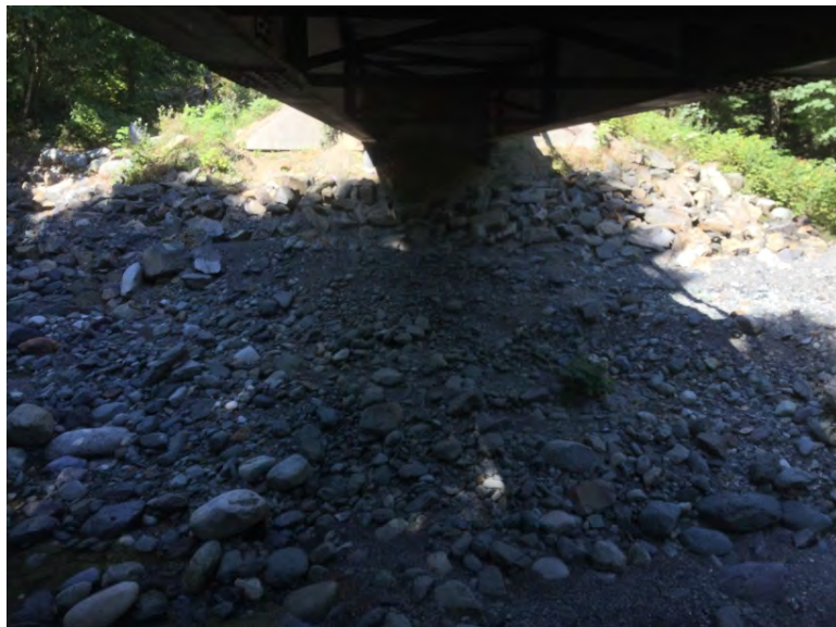
Left Bank Abutment when facing downstream
